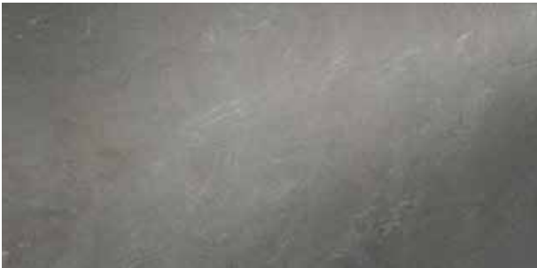
FULL SLAB VIEW
