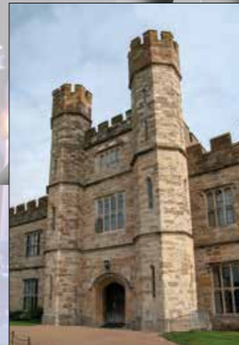
Leeds Castle, South Central Restoration
